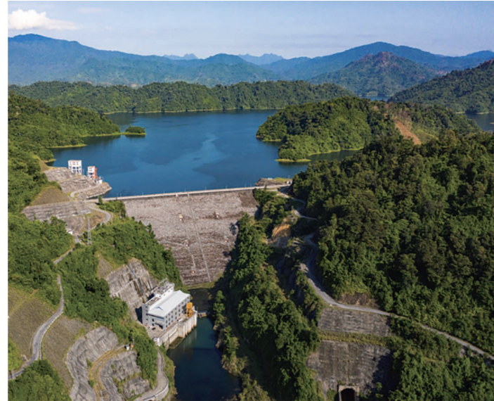
▲ 南立 1-2 水电站外景 An Exterior View of Nam Lik 1-2 Hydropower Station
