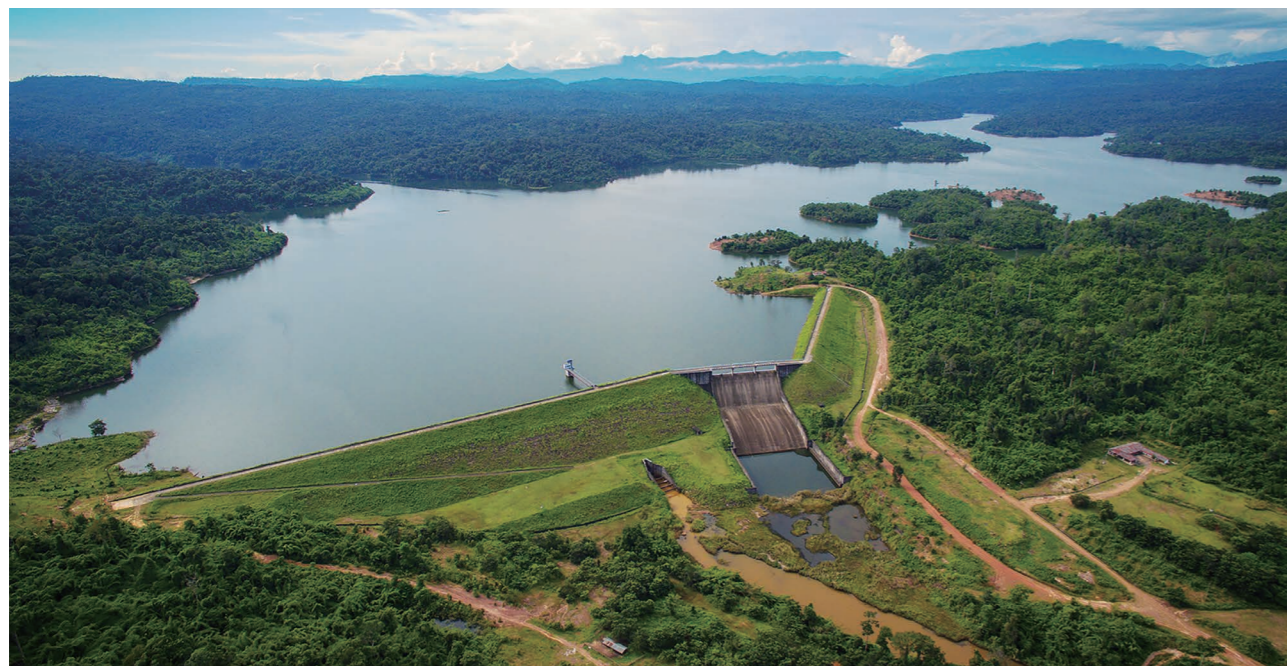
▲ 老挝南累克水电站 Nam Leuk Hydropower Station
