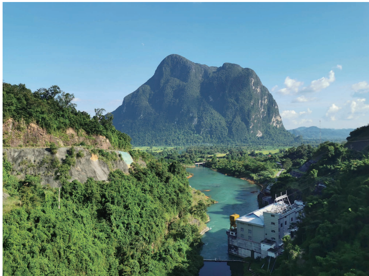
▲ 老挝南立 1-2 水电站发电厂房 Power House of Nam Lik 1-2 Hydropower Station
